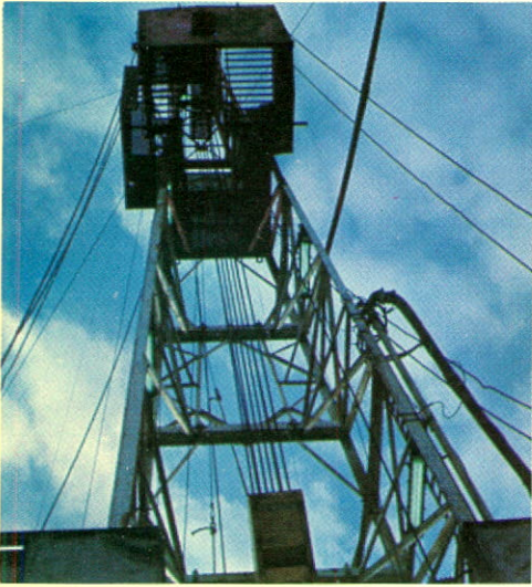
Derrick, Commonwealth - Hi-Tower Rig No. 1.
