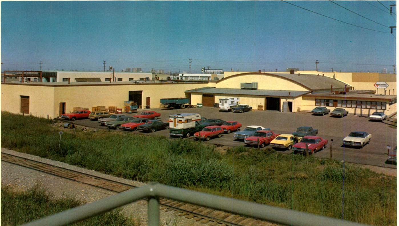
Flame-Master's new facilities in Edmonton, Alberta.
