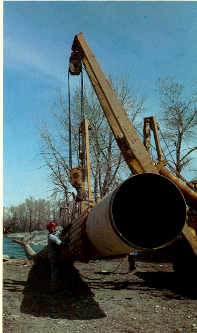
Wonderly and Kershaw laying 48" pipeline across the Bow River in Calgary.
