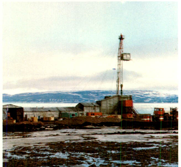
Commonwealth Hi-Tower Rig #2, on location in the Arctic.
