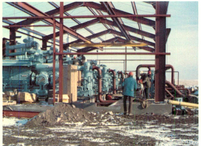
Compressor station during construction at Medicine Hat, Alberta.
