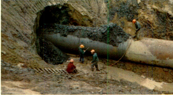
Water and power line contract in Alberta.
