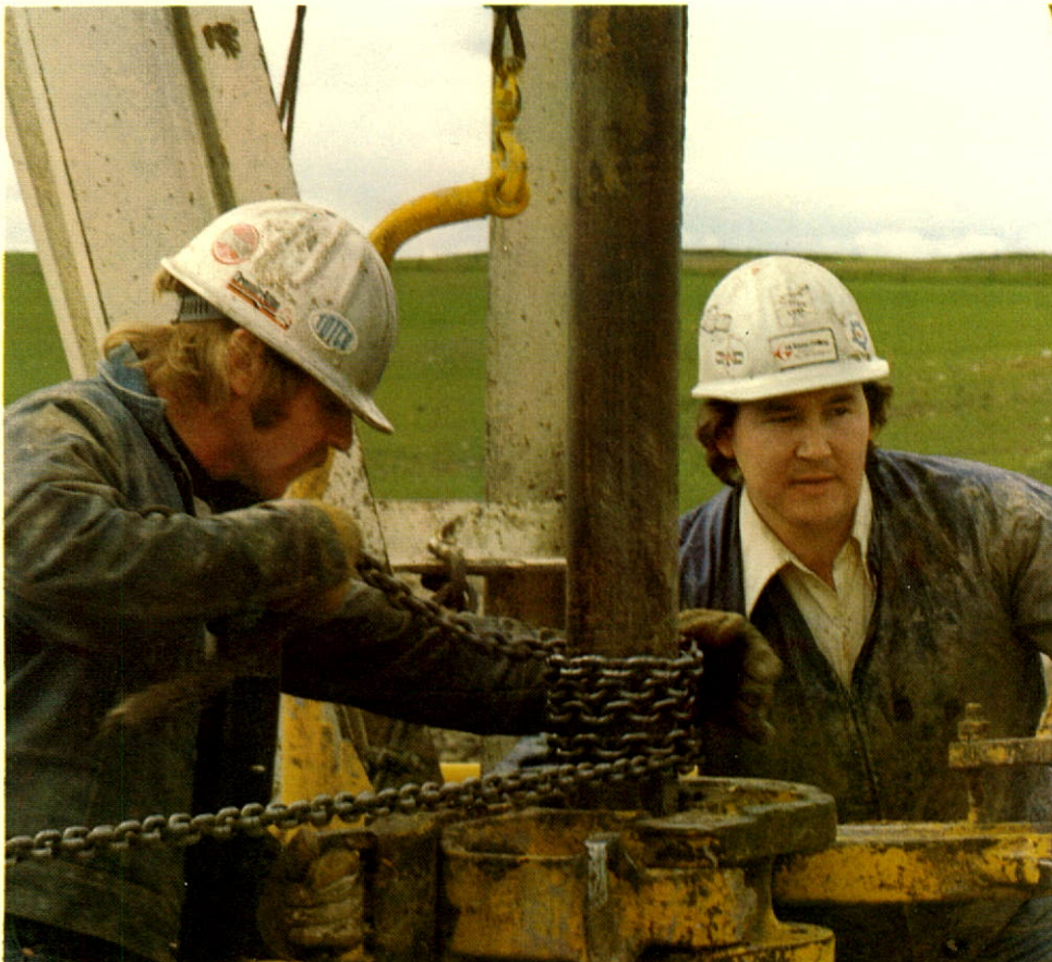
Hi-Tower rig and crew on location in southern Alberta.
