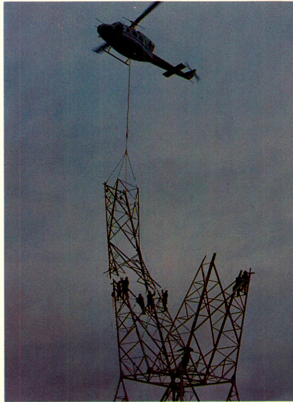
Bow Helicopters on a powerline installation contract in the lower mainland of British Columbia.
