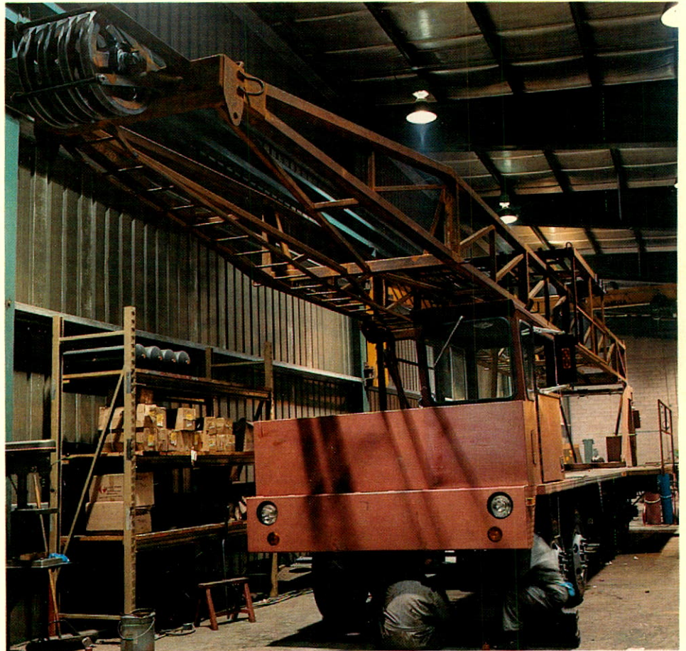
Assembling an oilfield service rig in Bow Valley's manufacturing plant in Vancouver, British Columbia.
