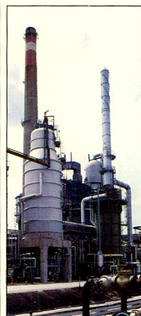
Petrosar's new vacuum distillation plant upgrades heavy fuel oil into vacuum gas oil, a more valuable product.
