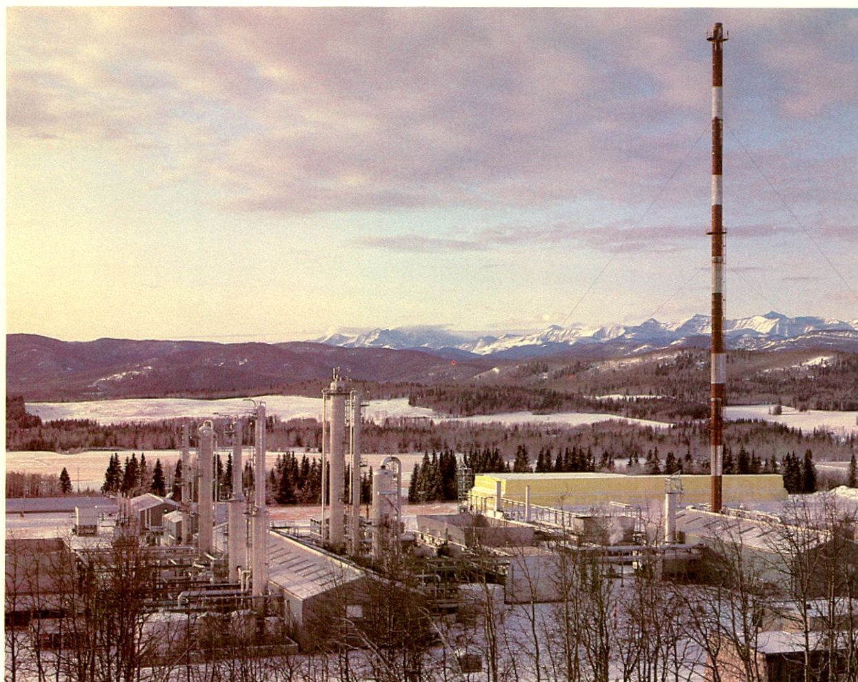
Quirk Creek natural gas plant, Alberta, Canada.
