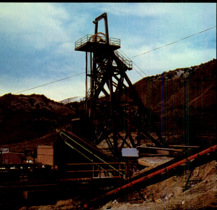
Headframe, Gooseberry Mine, Nevada.
