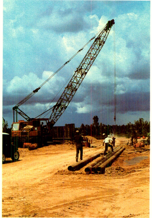
Pipeline construction, Ramba Field, South Sumatra.
