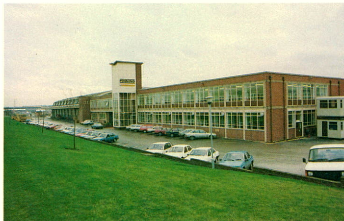
Main facility at Cannock, near Birmingham, is centre of operations for merged UK dealerships now known as Finning Limited.
