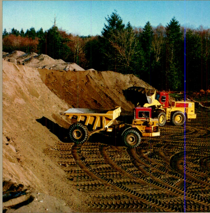
Caterpillar wheel loader fills DJB truck for construction of approaches to new Annacis bridge.
