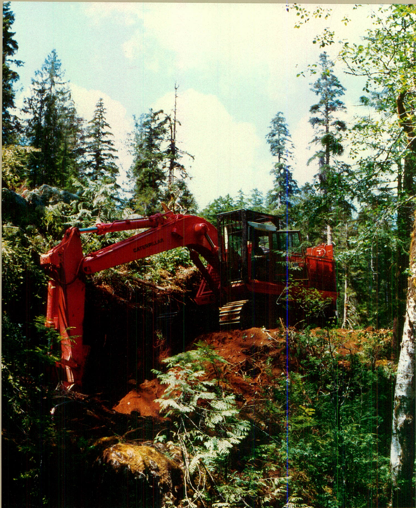
The 235 Roadbuilder, a Caterpillar hydraulic excavator modified by Finning, achieved excellent sales as the forest industry again was the major contributor to machine volume.
