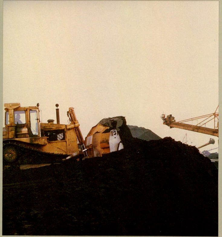
Cat D8L Tractor can push 27 tons of coal in one pass at deepsea terminal at Roberts Bank.
