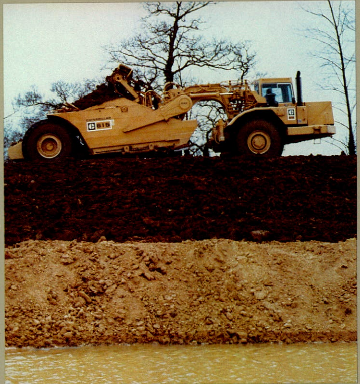
Newly-introduced 615 self-loading scraper is used in site stripping and land reclamation.
