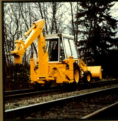
Trakhoe developed from JCB 1550 backhoe replaces worn rail ties.
