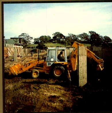
New JCB 1400 backhoe loader excavates basement in Victoria.
