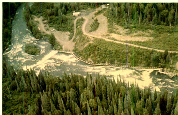
Meziadin Fishway on the Nass River, built in 1966, has enabled good numbers of fish to move beyond the blockages to the upper reaches of the river. (F. Dickson)
