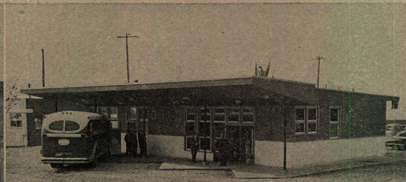
New bus depot and office building at White Rock, B. C.
