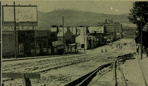
Street car tracks come up in Vancouver . . .
