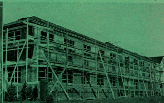
Extension to Oakridge Transit Centre under way
