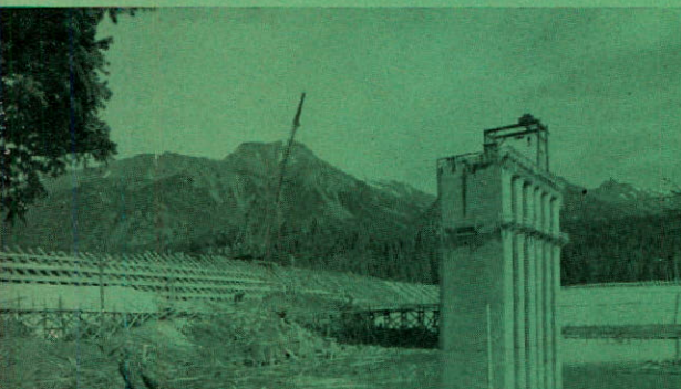
La Joie Storage Dam raised 45 feet during 1950
