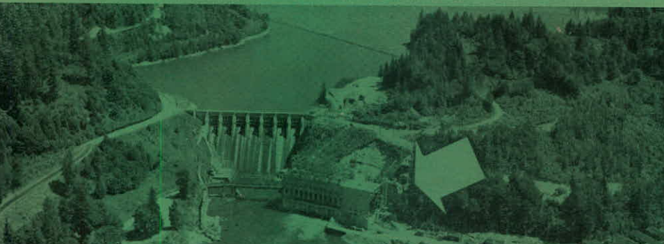
47,000 h.p. from the new third unit at Ruskin
