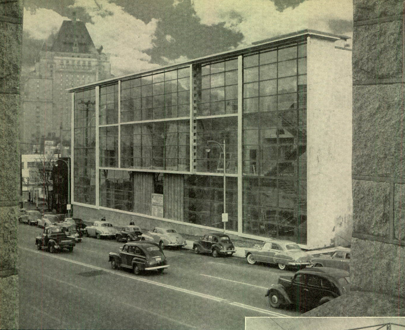
DAL GRAUER SUBSTATION nearing completion in downtown Vancouver is the latest of several large post-war installations of substation equipment in the metropolitan area.
