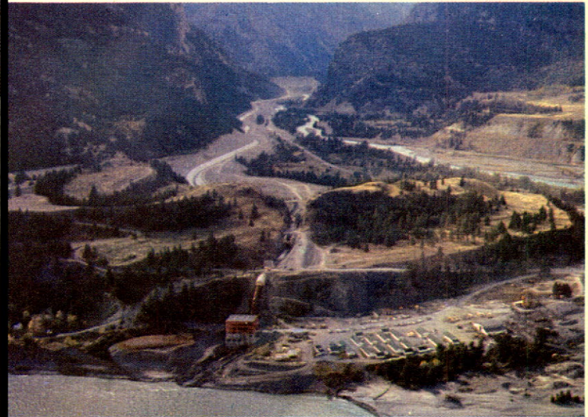
The water from Seton Lake (behind the mountains in the right background), which normally flows through Cayoosh Creek on the right, will be channeled by a canal to the generating station on the Fraser River 1½ miles south of Lillooet, B.C.
