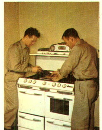
Over 120,000 customers' appliances were adjusted to use natural gas instead of manufactured gas.
