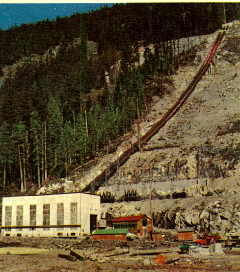
The Cheakamus development can produce 140,000 kw. Water diverted through a 6¾ mile tunnel is dropped through penstocks 1,700 feet long to the powerhouse on Squamish River.
