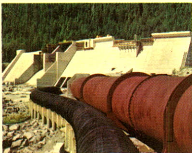
This dam stores water for the new Clowhom hydro-electric station, which can produce 30,000 kw, 10 times the capacity of the small, two-unit plant it replaced.
