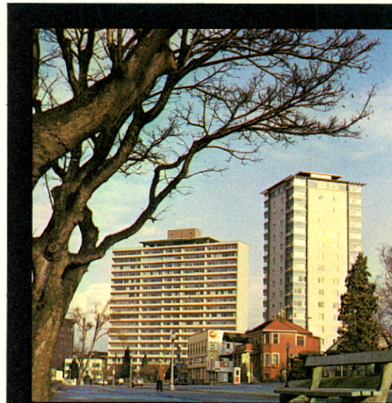
59 apartment buildings, including the two above, began using gas for heating and other purposes in 1959. In all, 165 large-volume customers were connected in 1959, including the new medical building seen below.
