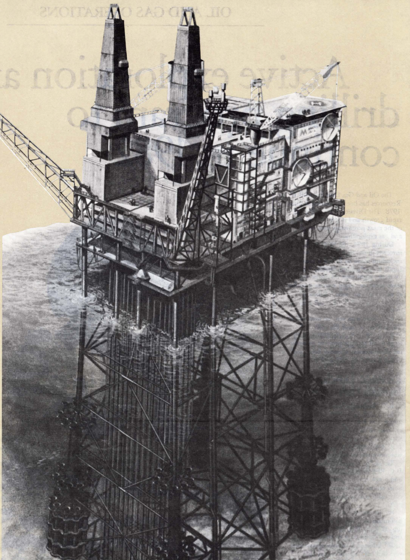
Mammoth production platform now under construction in Europe will be capable of producing 100,000 barrels of oil daily from the South Brae field in the North Sea. Artist's conception shows how structure will be anchored to the seabed, about 250 kilometers from the coast of Scotland.
