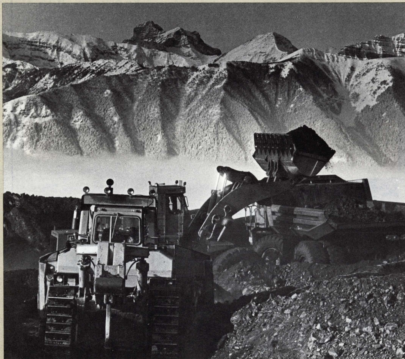
Giant front-end loader at work at the new Greenhills Mine.
