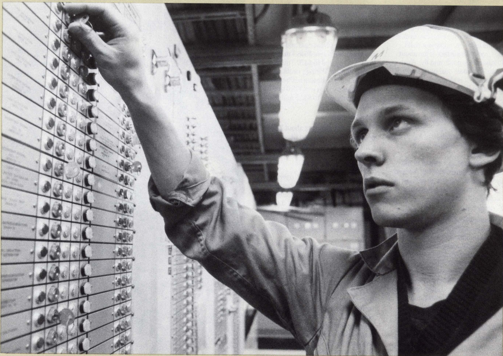
Flow of oil and natural gas liquids from the South Brae production platform is monitored by highly skilled employees using state of the art technology.
