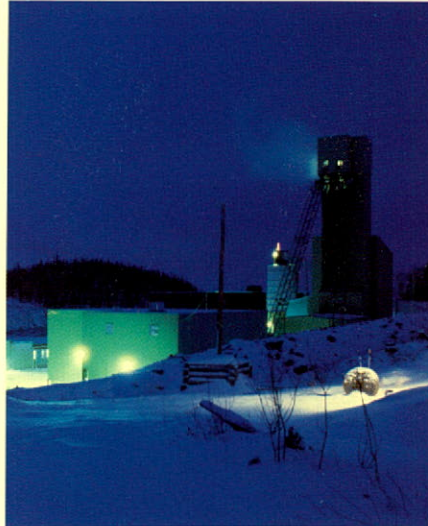
Winston Lake - headframe and mining plant
