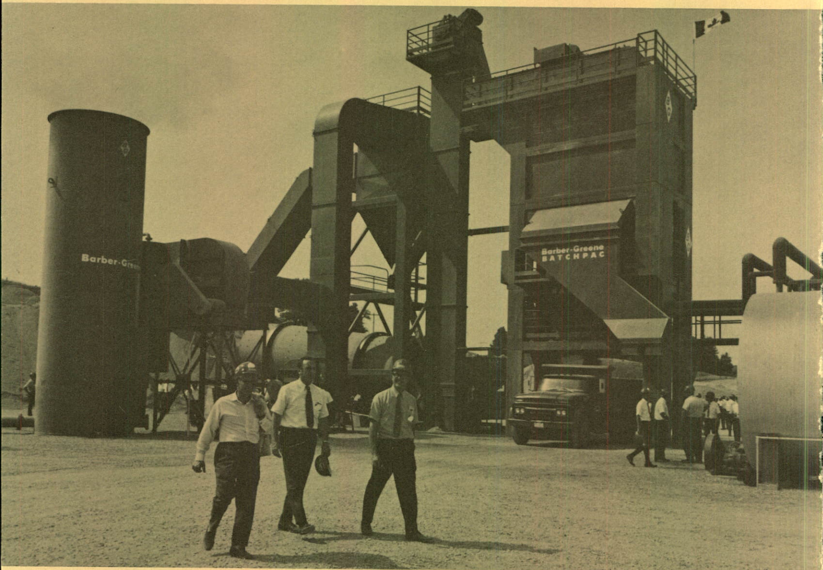
Blacktop Construction's 300 tons per hour asphalt plant near Kitchener.
