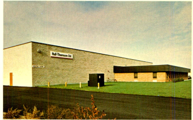
Hull-Thomson's new facility in Windsor, Ontario
