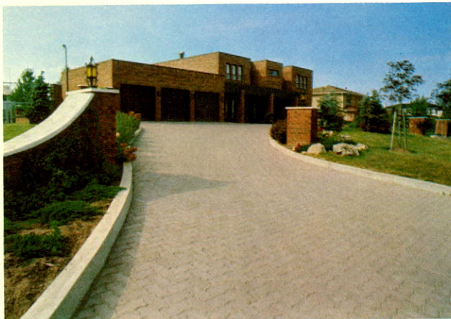
Interlocking paving brick—a new market for synthetic iron oxides produced by Northern Pigment.
