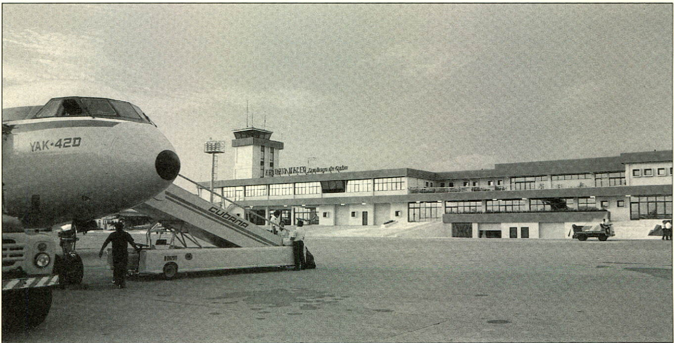
▲ A contract for the completion of the interior and equipment installation at Antonio Maceo Airport, Santiago de Cuba, was awarded by CCC to Regor International Inc., of Montreal, Quebec.
