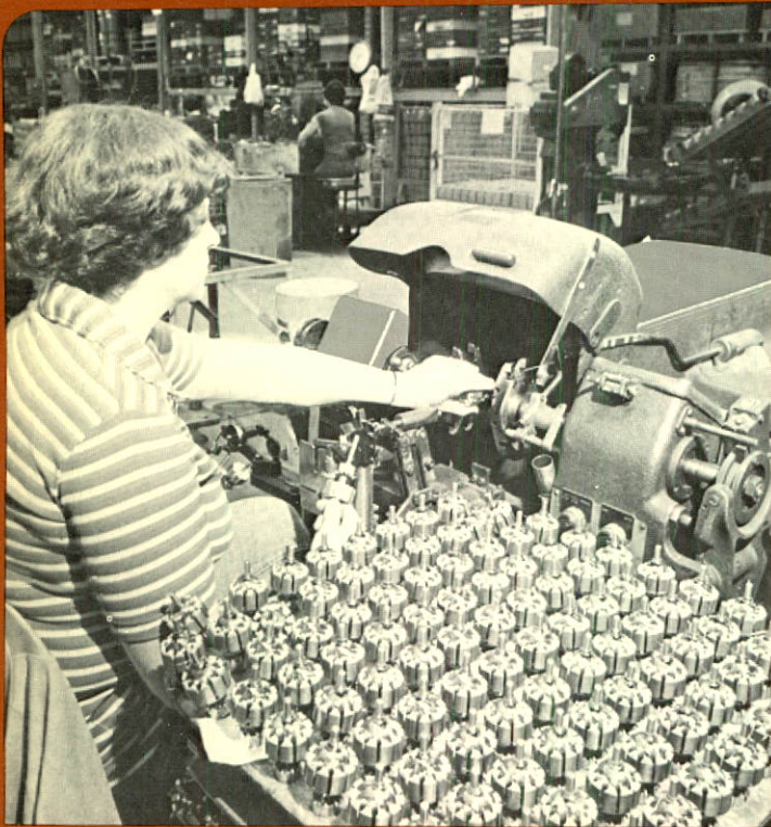
Semi-automatic armature winding for D.C. motors
