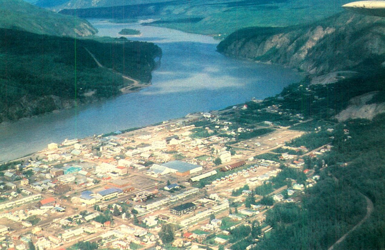
Dawson, Yukon, and other northern communities have reduced the cost of installing water and sewer lines by employing insulated polyethylene piping systems developed by the Company.
