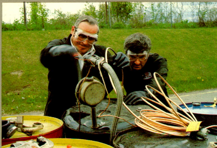
A Chemical Emergency Response Team at Maitland Works, part of a national program established by the chemical industry, responds to regional transportation incidents. Maitland team members Gil Laframboise, left, and John Montgomery remove volatile liquid from damaged drums following a transportation accident.
