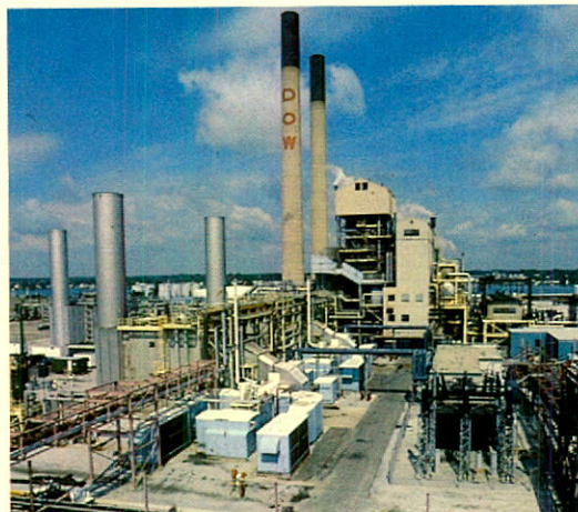
Power plant, Sarnia Division: generating our own electricity and steam from natural gas fired turbines. Co-generation technology yields energy efficiency in 80 percent range, double conventional methods.
