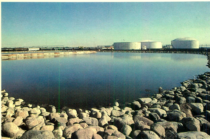
Process water treatment and storage pond on Fort Saskatchewan plant site, where millions of liters are purified, recycled rather than becoming a waste material.
