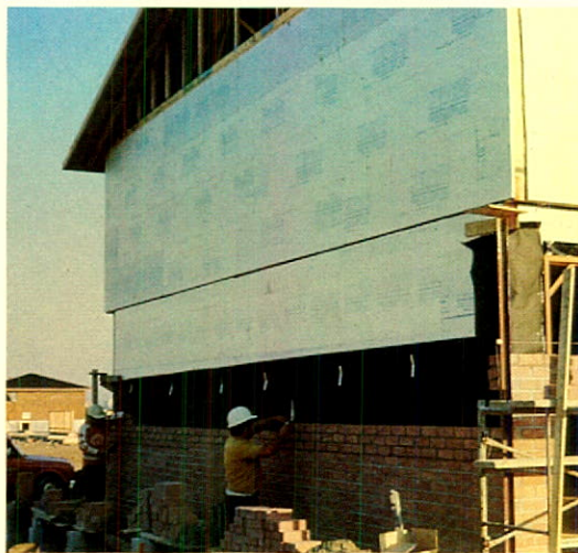
"Blue blanket" of Styrofoam SM insulating sheathing ensures fuel conservation in new or retrofit projects.
