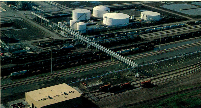
Marshalling yard with 25 km trackage on our Fort Saskatchewan site permits train make-up for greater safety, improved efficiency.
