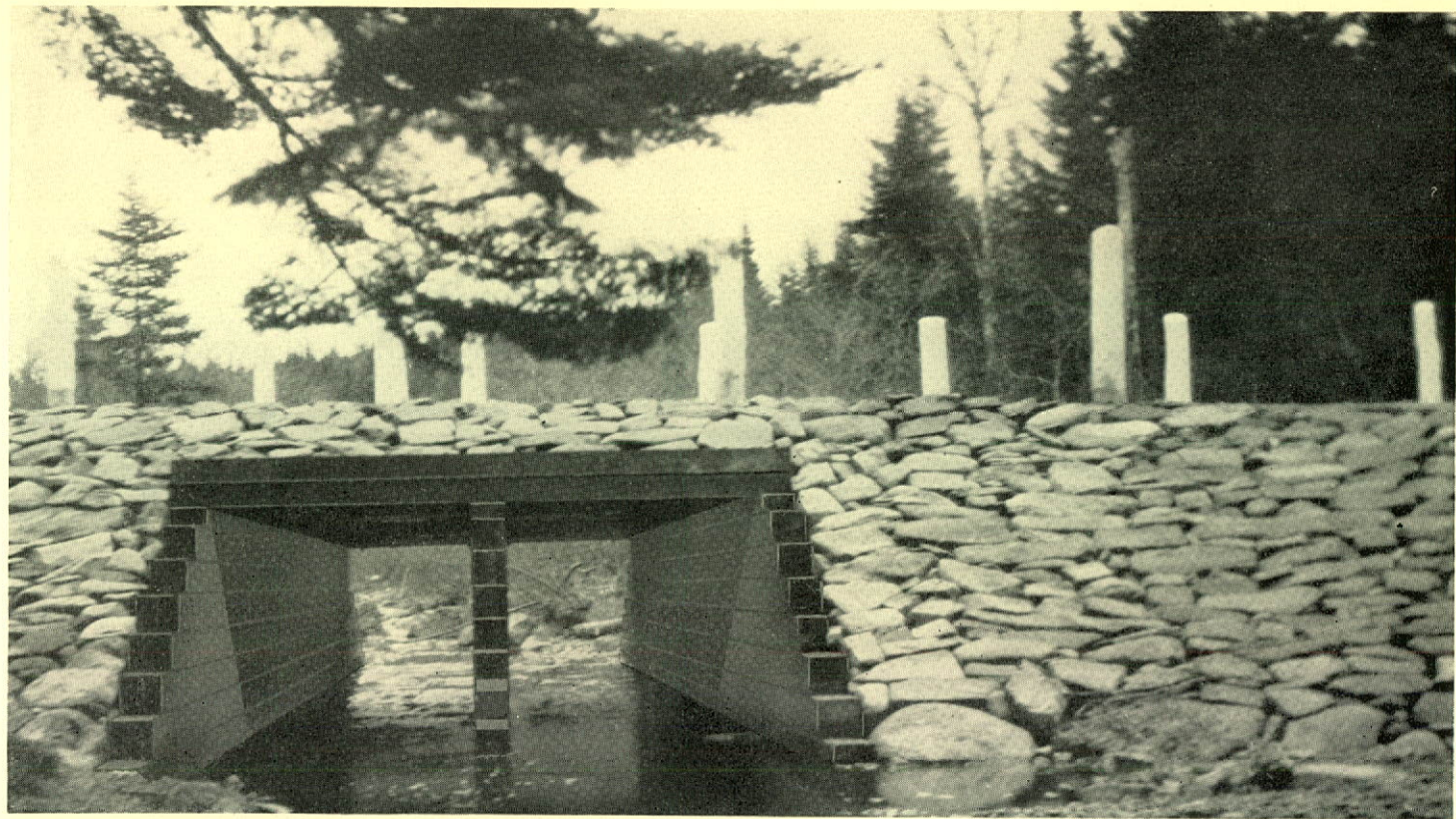
CREOSOTED LAMINATED TIMBER CULVERT INSTALLED IN NEW BRUNSWICK.
