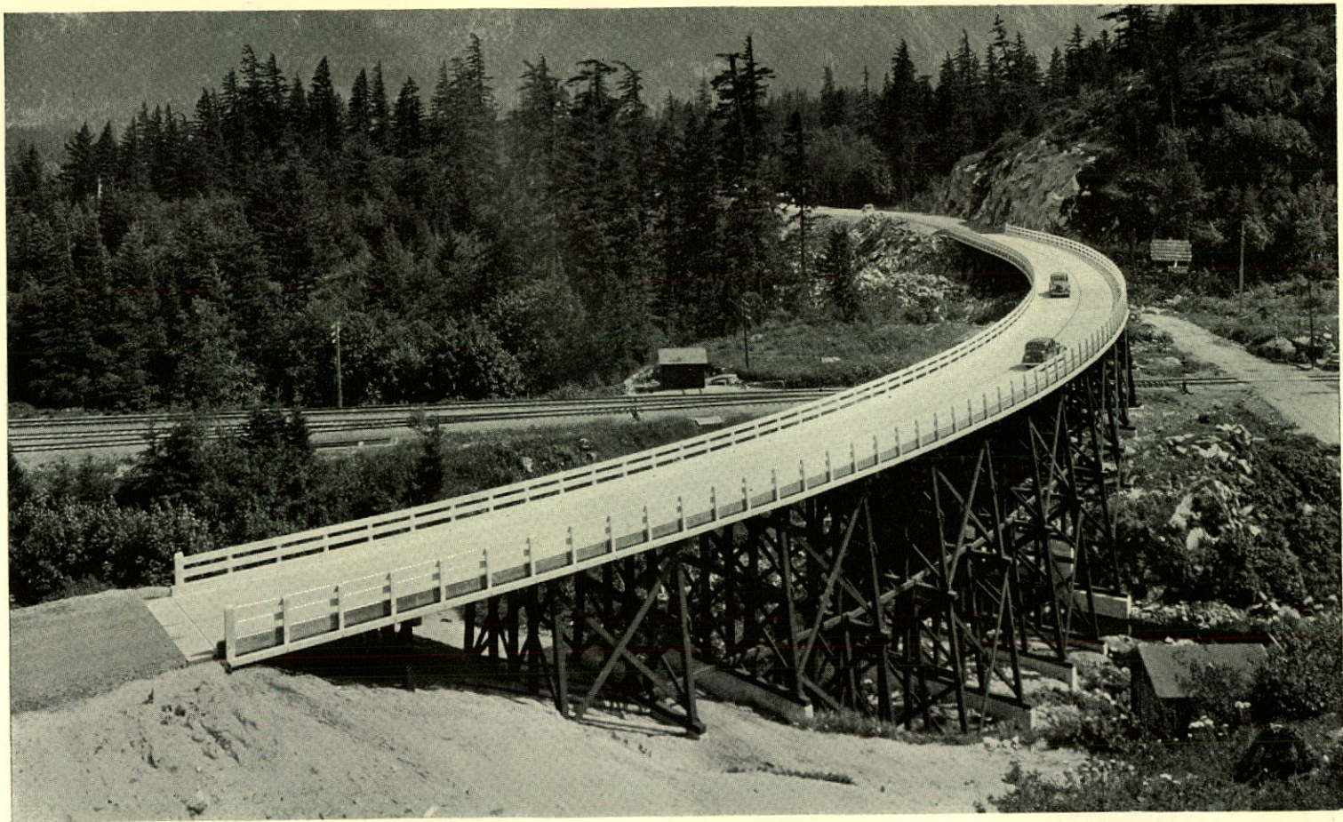
OVERHEAD CROSSING—OVER C.P.R. MAIN LINE AT HAIG, B.C.
