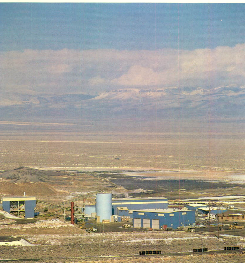
General view of the Pinson milling and maintenance facilities in Nevada.
