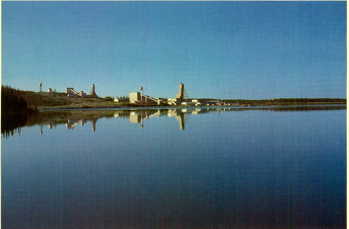
The Mill and Original Mine at sunrise.
