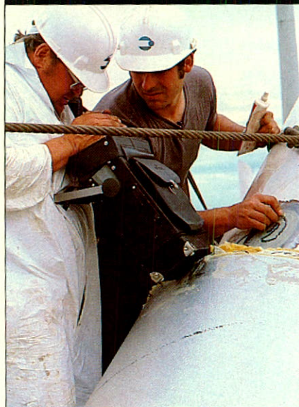
Right: Installation of new pipeline strainer. Station 17, Regina, Saskatchewan.
