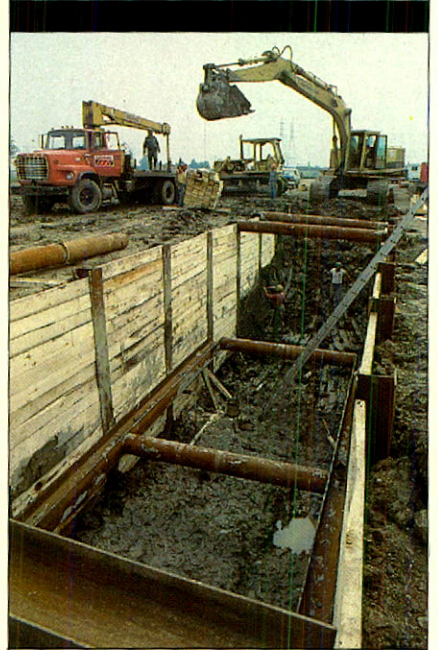
Right: Welder making a connection on 406 mm pipe replacement, TQM line near St. Lazare, Quebec.
