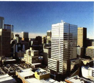
TransCanada's Calgary office is located at the hub of Canada's oil and gas industry.
