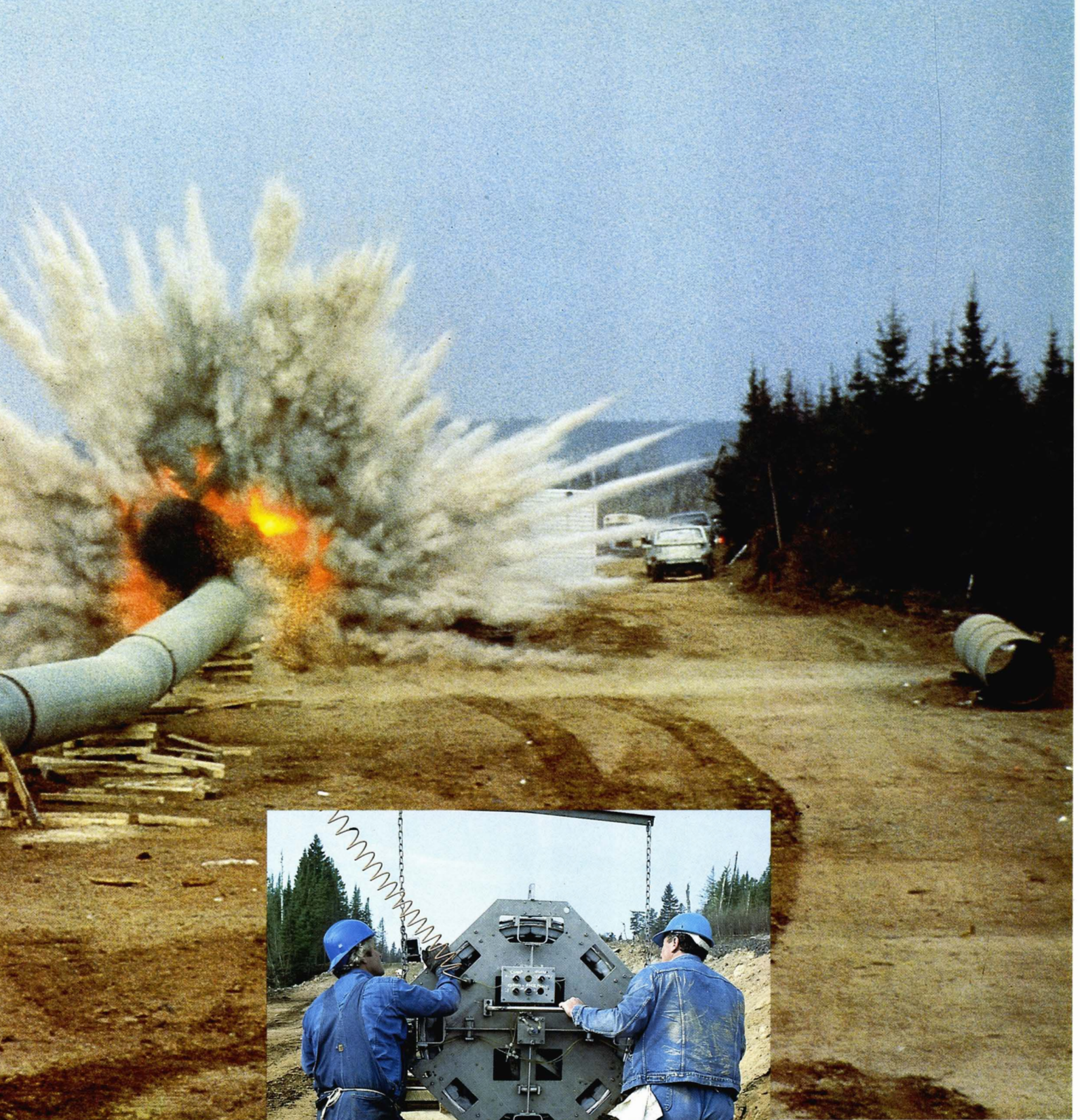
In 1984, the company was the first to test the use of explosives in welding a large diameter natural gas pipeline. The successful test was conducted on a 6.1 kilometre section of line near Thunder Bay, Ontario.
