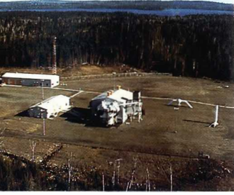
Station 69, near Thunder Bay, Ontario, is one of the company's automated compressor stations.
