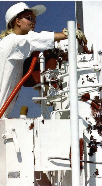
Careful maintenance of all equipment on the pipeline is a vital part of service responsibility. At Station 25 at Moosomin, Saskatchewan, valves are sandblasted and repainted.
