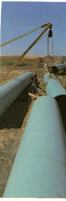
Pipe is strung along the right-of-way in preparation for welding.
