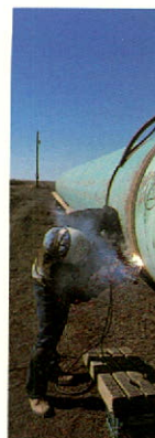
A welder completes a tie-in, linking long sections of pipe together.
