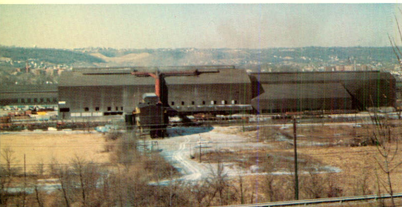
At Wilder, Ky.—the dust you see coming from our melt shop will soon be controlled by our new bag house shown in the foreground.
