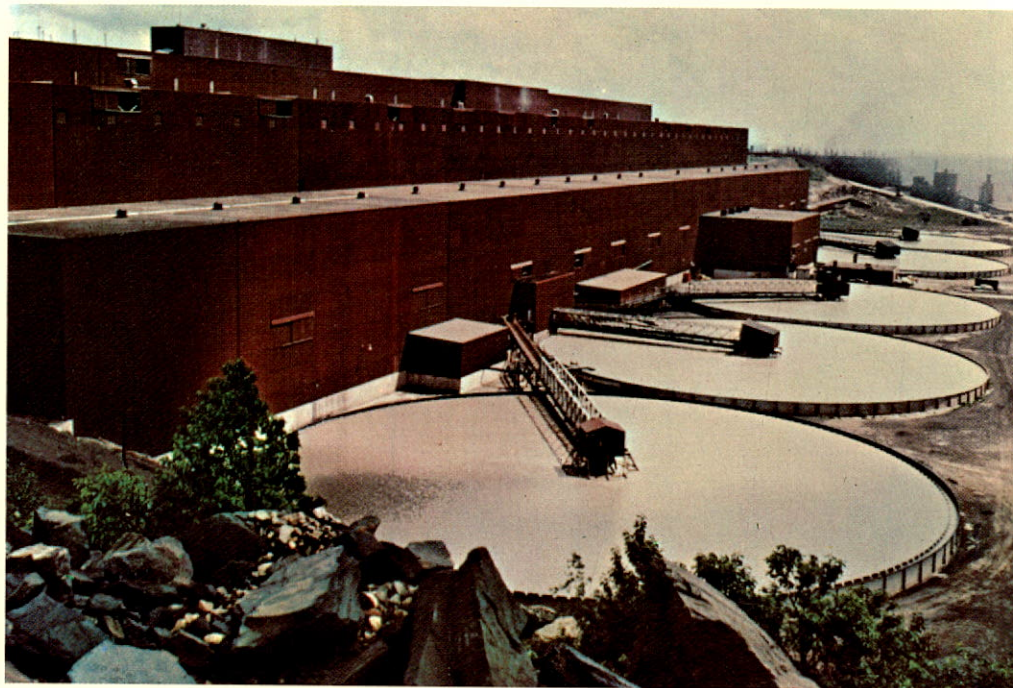
Top photo: Shows water pollution control clarifiers at the Erie Mining plant in Minnesota. Bottom photo shows inside of Erie ball mill where taconite ore is ground into powder before being pelletized.
