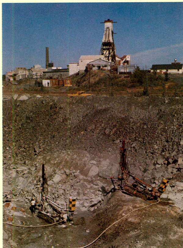
Open pit work — C-Shaft headframe in background
