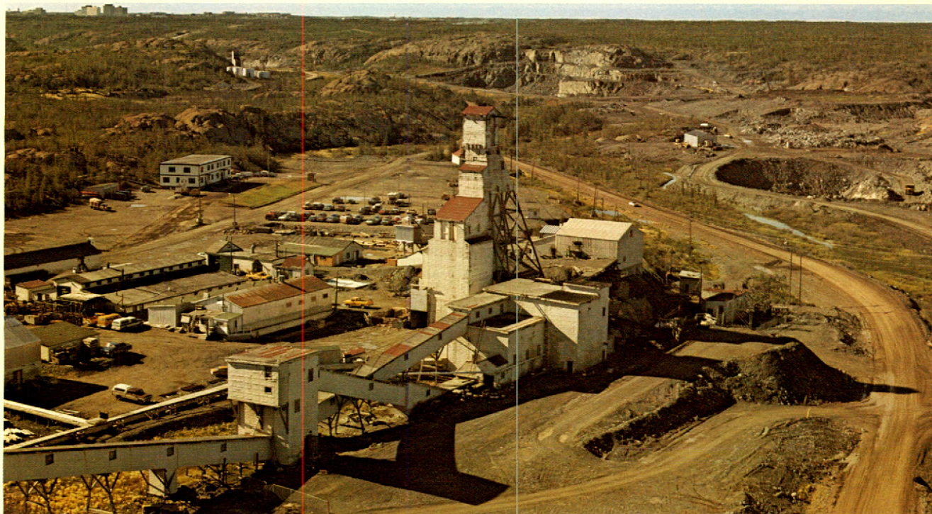
C-Shaft Headframe with C-1 pit in foreground and A-1 pit in background.
