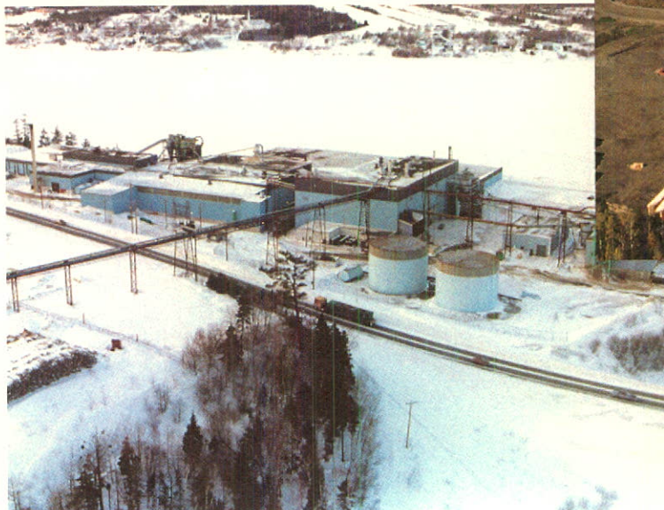
Part of the Atlantic Waferboard Inc. plant on the banks of the Miramichi.
