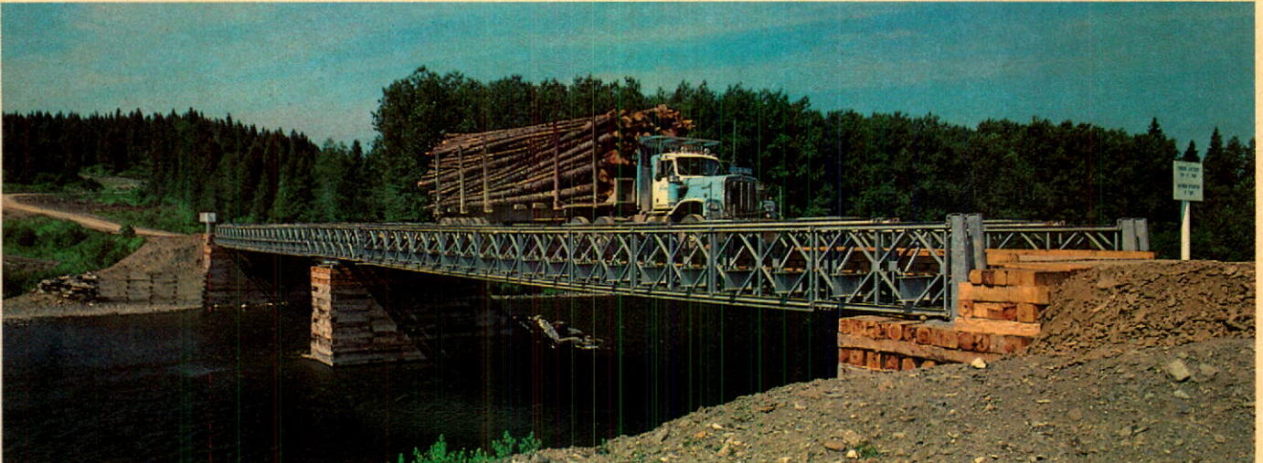
Over 200 ft. long, this newly constructed two-span bridge over the Kedgwick River improves access to our forest resources.
