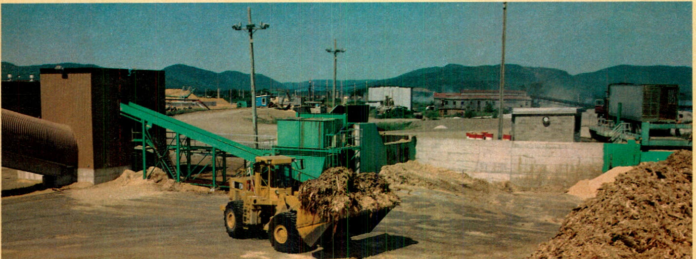
Part of the biomass operation used to attain over 85% self-sufficiency in energy and power at Atholville.
