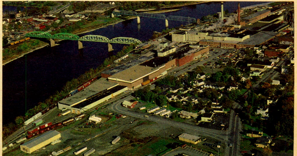
Today's huge industrial complex at Madawaska with twelve major machine operations.
