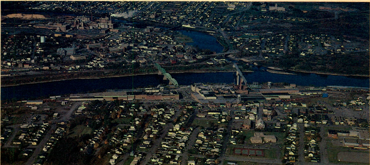
Edmundston (top) and Madawaska (bottom) Mills are interconnected with pulp lines and steam line (right) for more efficient operation.
