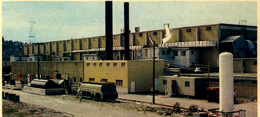
Island Paper Mills Limited plant on Annacis Island, B.C.
