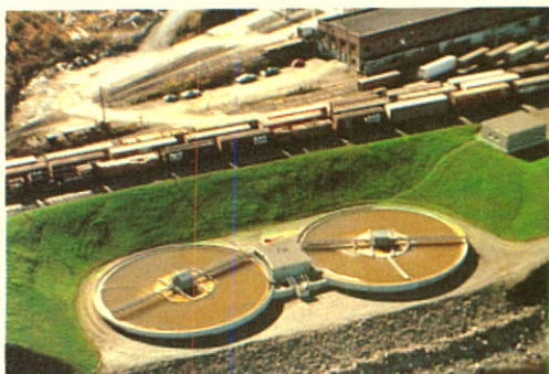
Twin clarifiers - Madawaska
