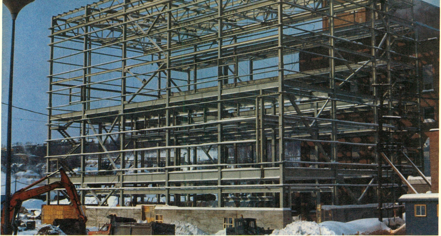
Construction of new washing and screening building
