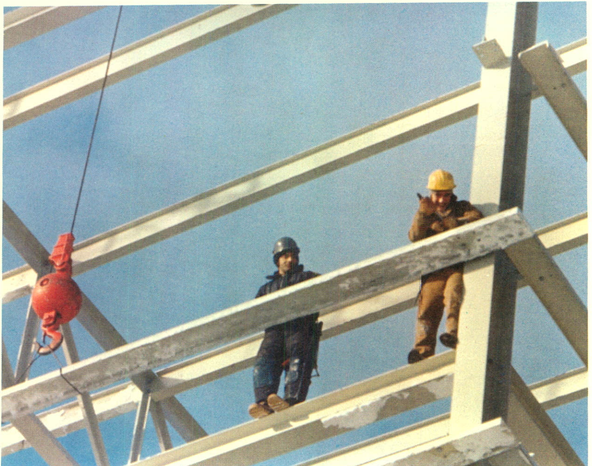
Steel riggers at work
