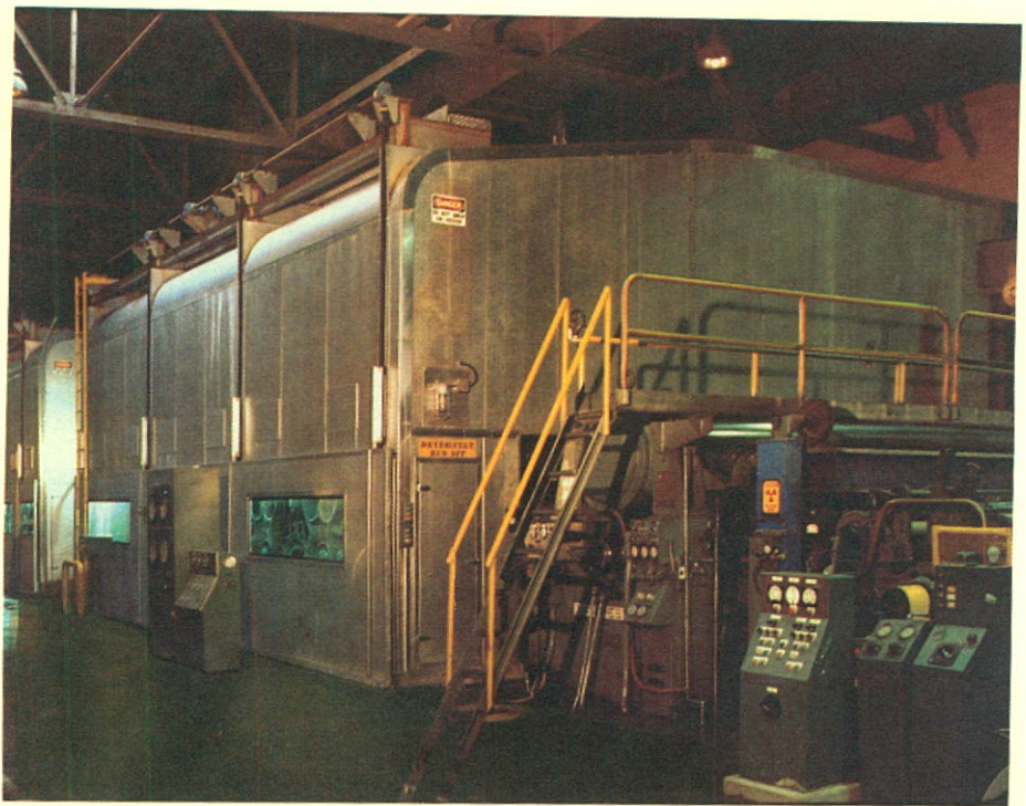
New dryer hood - No. 3 Paper Machine
