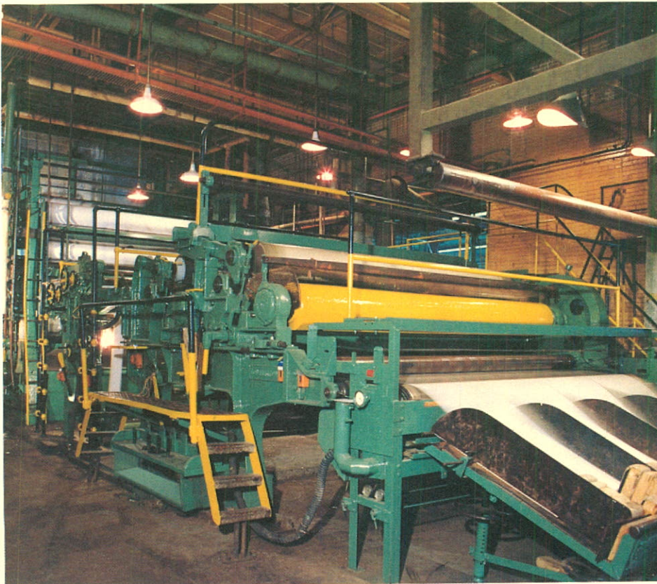
Newly painted boxboard machine
