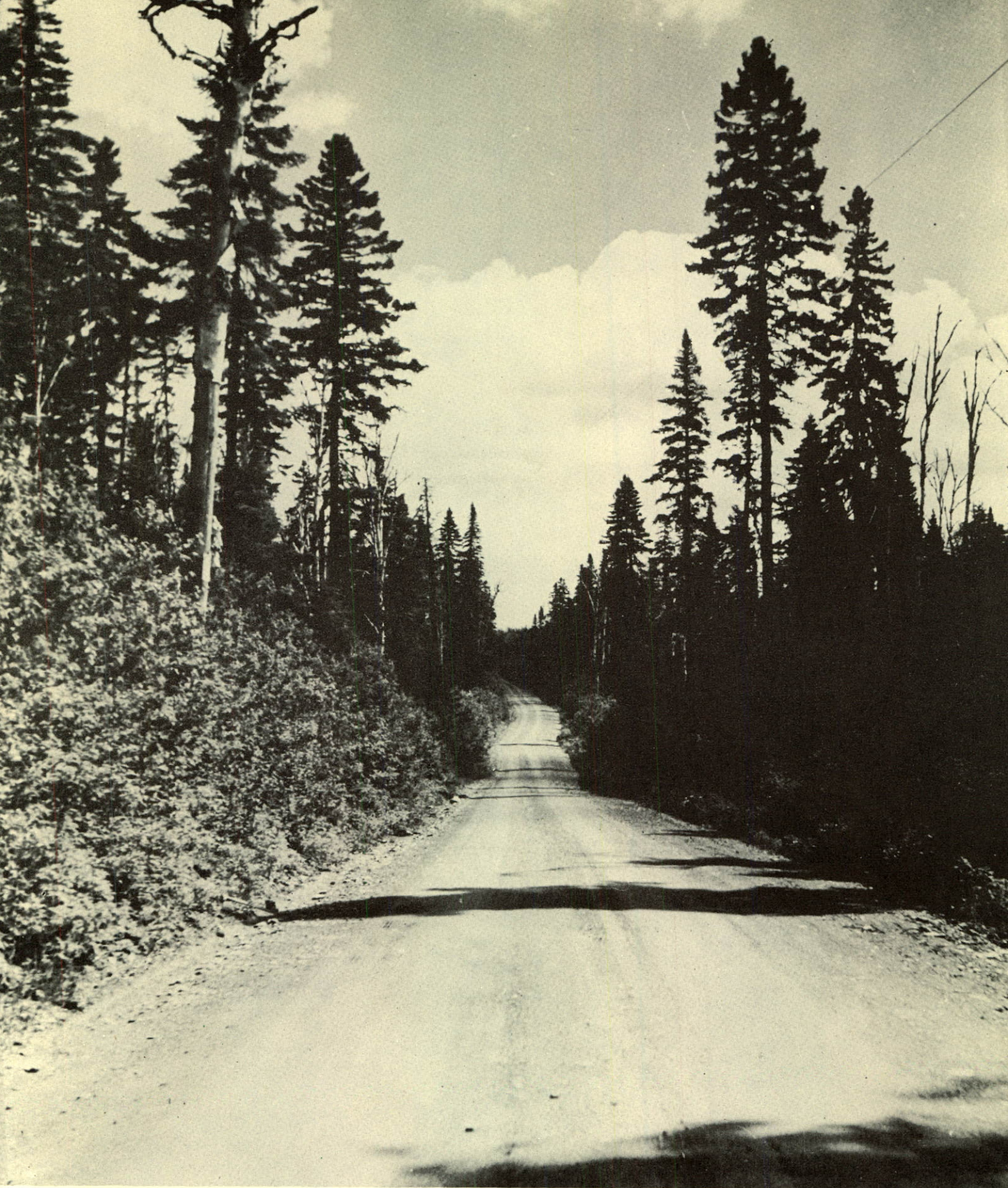
Typical of many such roads, built for the development and management of timber lands and limits, is this view of the Pemouet Forest Road on Green River Drainage.
