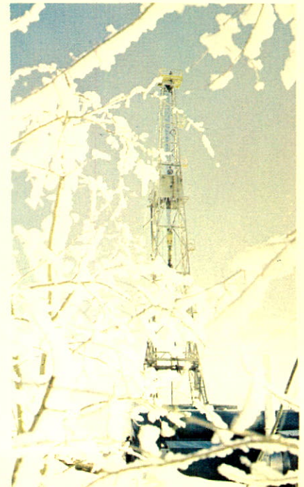
Winter drilling in northeast British Columbia.
