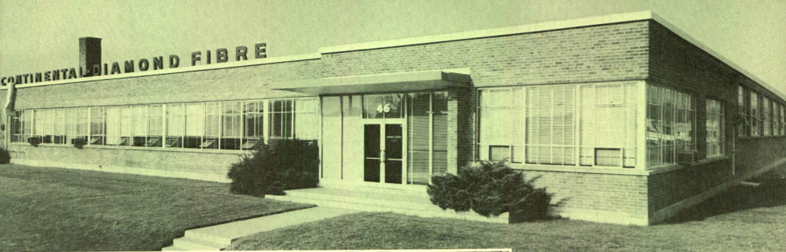
Plant of Continental-Diamond Fibre Division, The Arborite Company Limited, Toronto, Ont.
