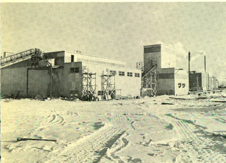
Hardwood Woodroom at Cornwall Division of Howard Smith. Can bark, chip and screen up to a capacity of 300 tons a day.
