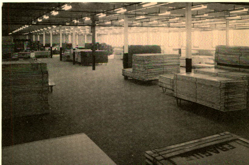
A section of the Extension to the plant of The Arborite Company Limited, LaSalle, Quebec
